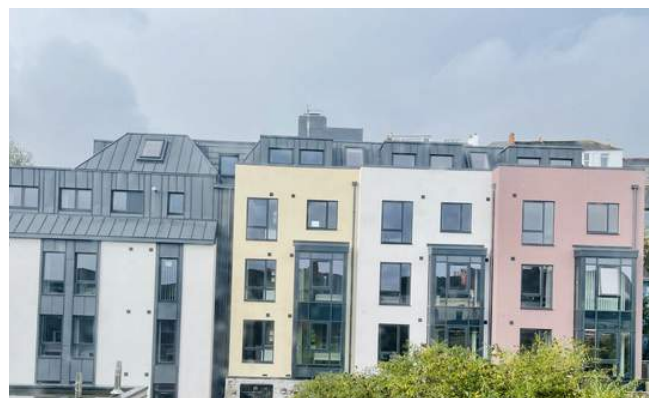
112 single-occupancy studio apartments in a PBSA scheme in Falmouth, co-financed by ASK and OakNorth Bank
