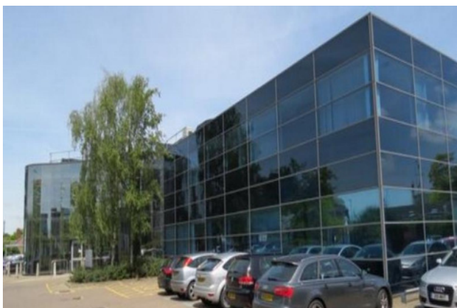
A Cambridge office building acquired for conversion to lab space, funded by ASK
